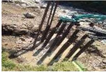
**Gambar 8. Pengecoran bore pile**
